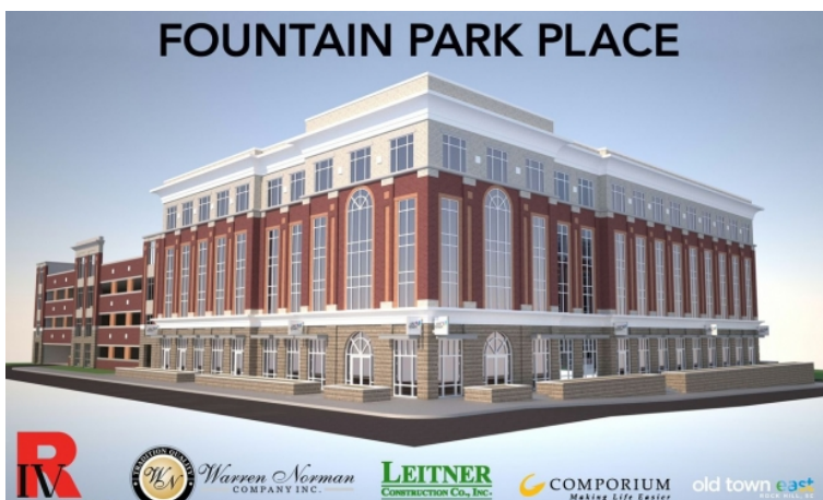
Rendering of Fountain Park Place, under construction in Old Town East.
